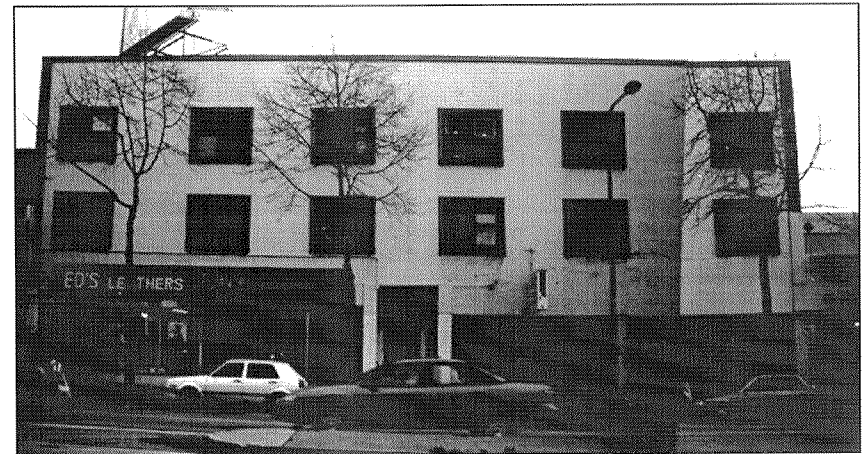
Some facades that are run-down and need to be repaired and painted create an impression that the University Avenue Corridor is a dying commercial strip.
