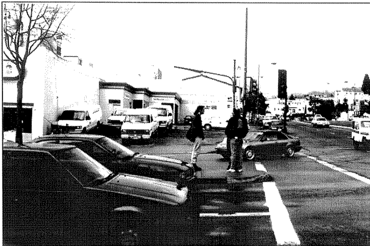
Enhanced streetscapes will help improve the safety and economic vitality of the Avenue and enliven pedestrian activity.
