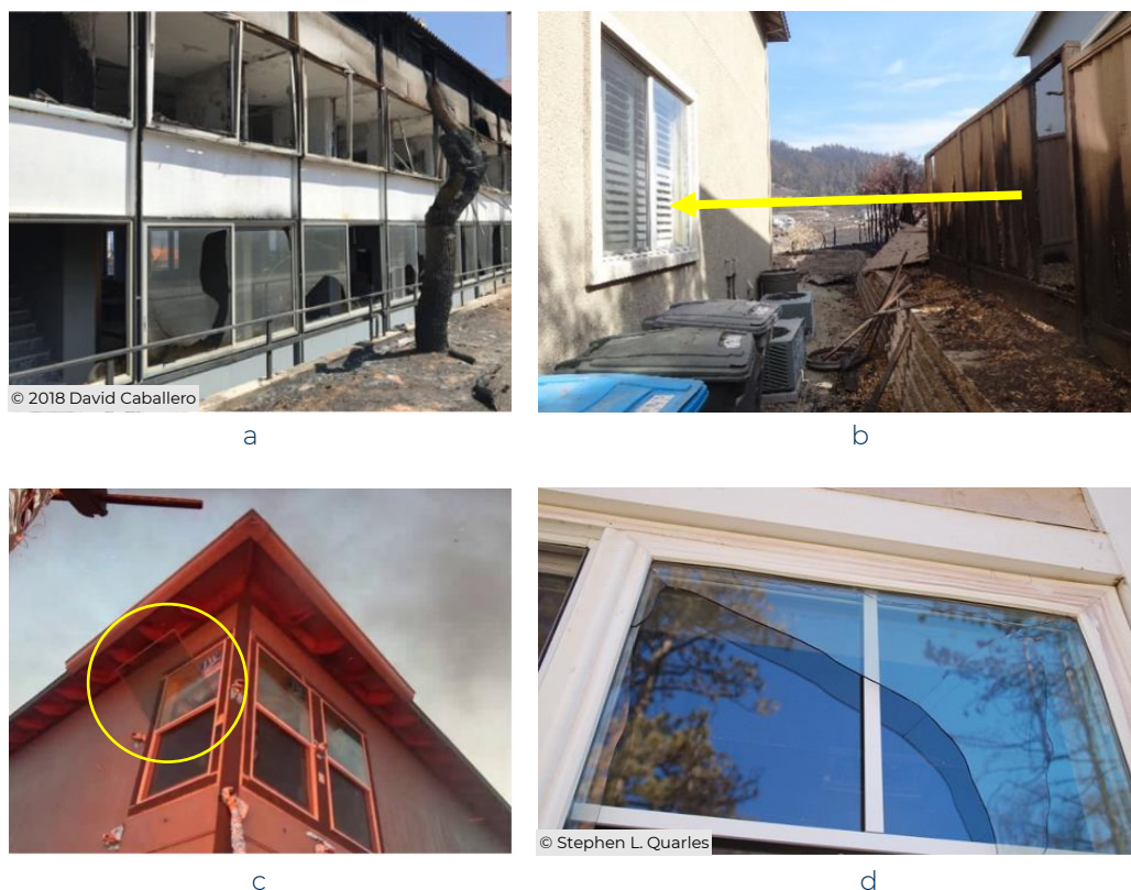
Figure 13. Vulnerability of windows: (a) glazing collapsed in Neos Voutzas-Mati, Greece (2018) due to the combustion of a pine tree ( Peñaloza et al., 2021 ), used with permission; (b) windows damaged by radiation from a burning fence about 10 ft away during the Glass Fire (2020) in Napa and Sonoma Counties, California, where the arrow indicates the direction of radiation; (c) the outer tempered pane of a window fell out during an IBHS full-scale test; (d) window damage following the Grass Valley Fire (2006) in San Bernardino County, California, due to a burning building about 40 ft away, documented by Stephen L. Quarles.
