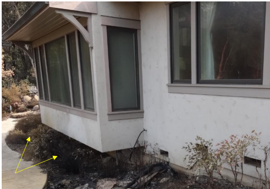
Figure 15. Heat trapped underneath bay windows caused the vegetation in this area to burn disproportionately to its surroundings during the Glass Fire (2020) in Napa and Sonoma Counties, California.
