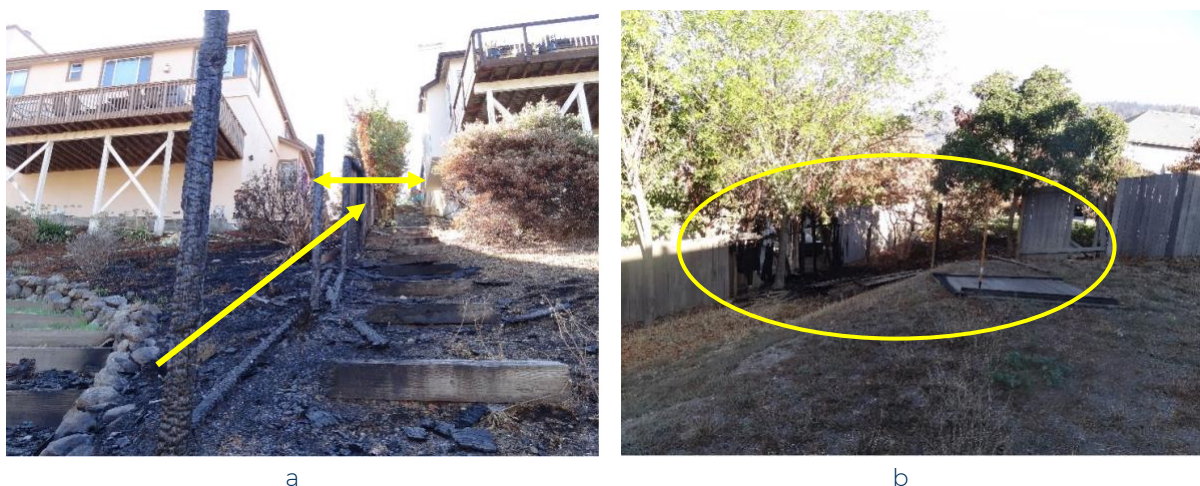
Figure 10. In the Glass Fire (2020) in Napa and Sonoma Counties, California, (a) a combustible fence provided a pathway for fire to spread uphill and damage both homes during fire, and (b) a wood fence spread fire and led to a cascade of damage (defended).
