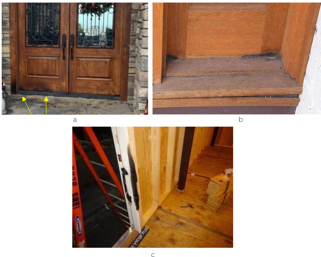
Figure 14. (a) Post-Marshall Fire (2021) investigation in Boulder County, Colorado, showing evidence of ignition from an accumulation of embers and debris at the base of the door; (b) Embers charred the threshold during the Victorian Bushfire (2009) in Australia ( Leonard, 2009 ), used with permission; (c) Embers ignite the door jamb at the IBHS Research Center.
