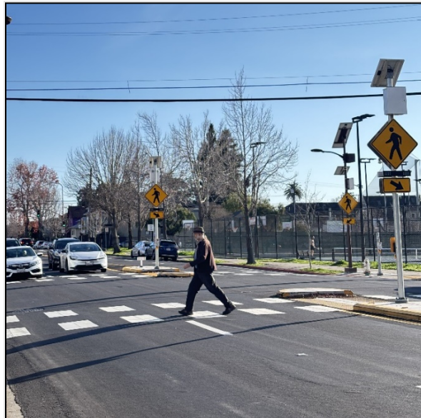
MLK Vision Zero Quick Build crosswalk improvements
