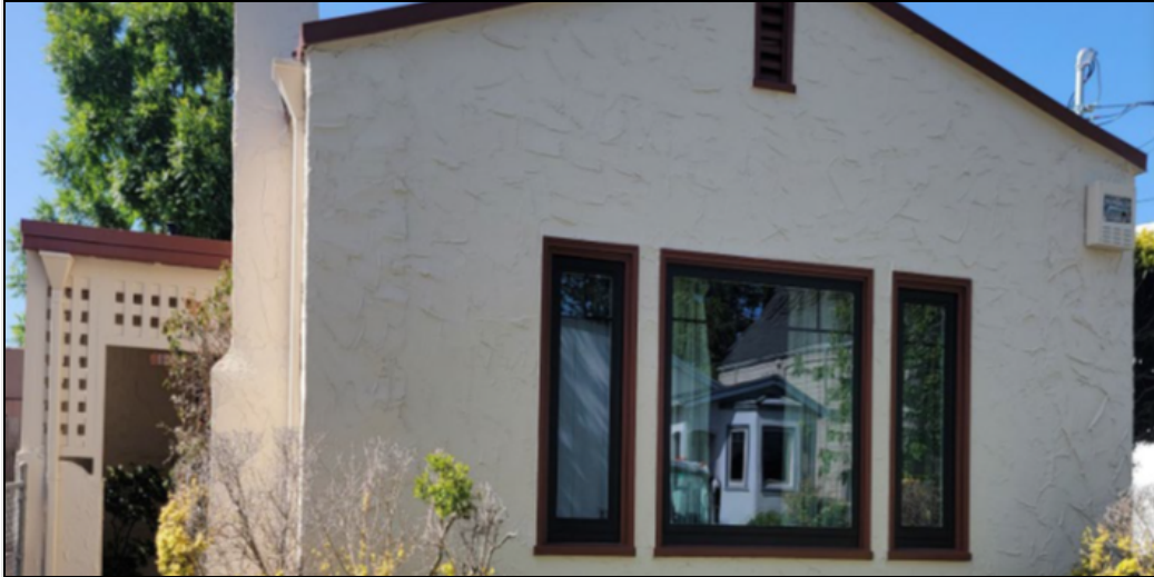
Berkeley home that received electrification upgrades through the Home Electrification Equity Project
