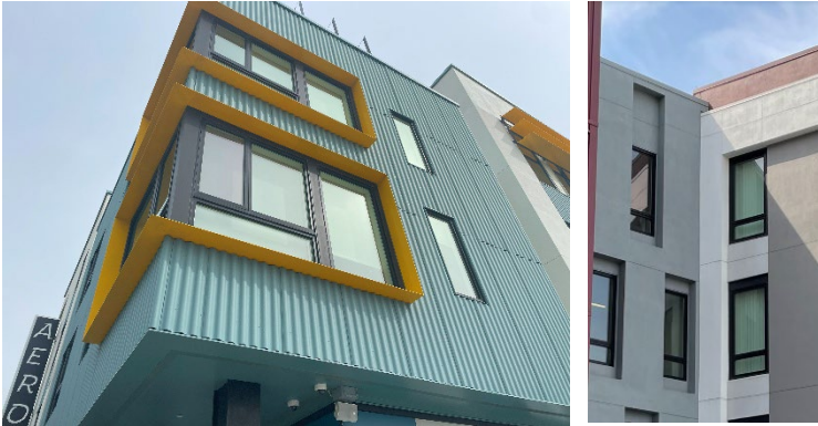
Framed windows and windows within a recess
