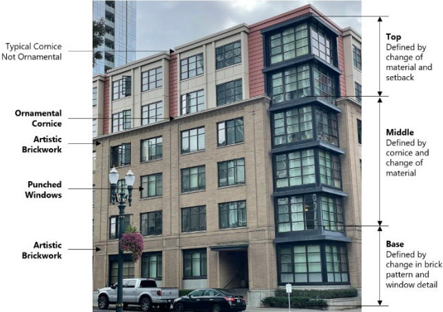
Diagram of Ornamental Façade. Source: Ashby BART West Lot Objective Design Standards (ODS)
