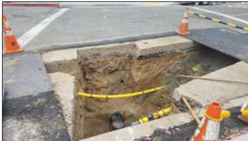
Figure 19. Utility trench at Adeline St and Harmon St. Note presence of trench sand, several layers of asphalt surface, and utilities 3-4 feet below ground surface.
