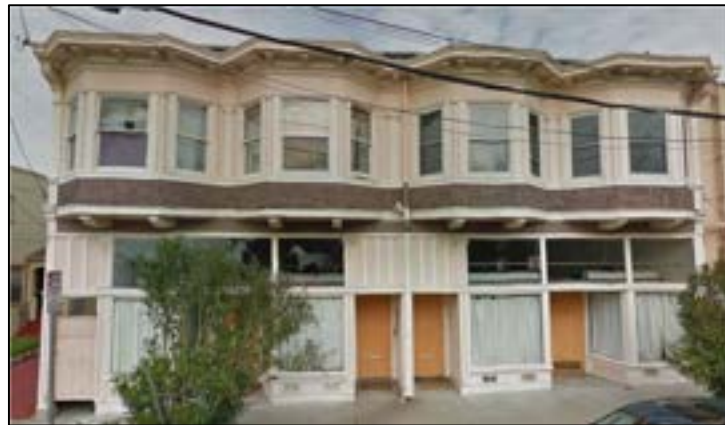
Figure 10. Mixed-use building at 1719-1721 63rd Street (built in 1907).
