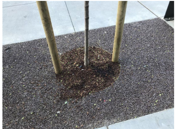
Figure 5.19 Flexible porous pavement in downtown Berkeley tree well
