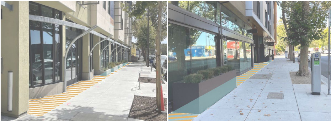
Figure 5.14 Examples of mixed-use residential developments with easement setbacks. Left: “Bloom Berkeley” 2747 San Pablo Avenue. Right: “The Jones” 2748 San Pablo Avenue.
