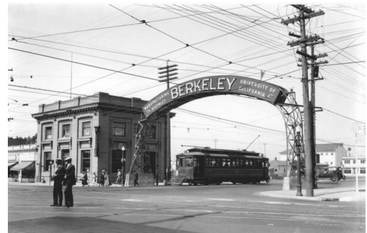
Figure 1.4 The Key System and Berkeley sign at San Pablo Avenue and University Avenue, ca. 1925. Source: Berkeley Public Library. Online Archive of California
