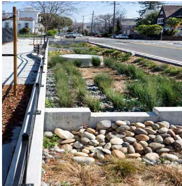
Green infrastructure installation at Woolsey Street
