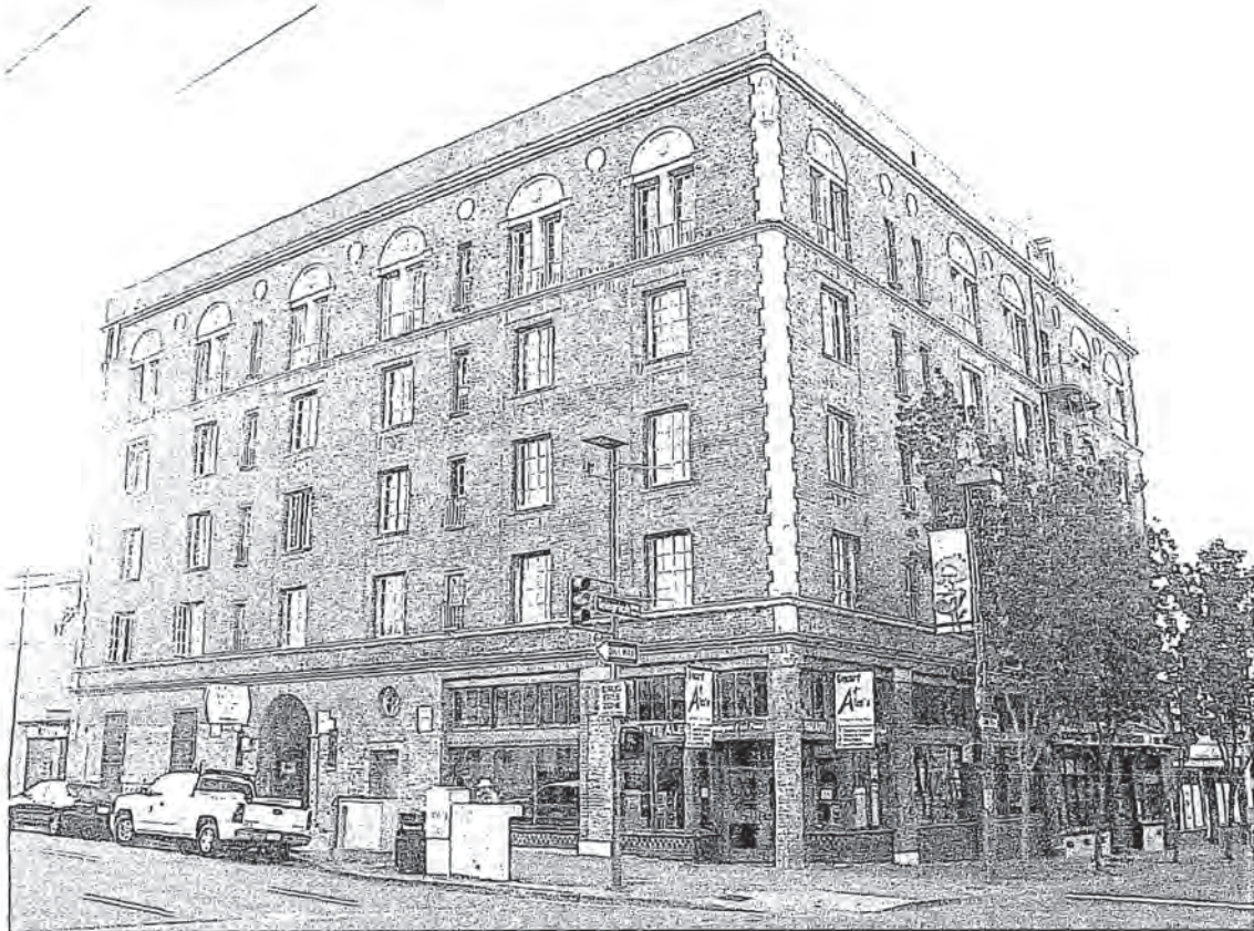
Photo 1. August 2007. The Cambridge Apartments, looking southeast.
