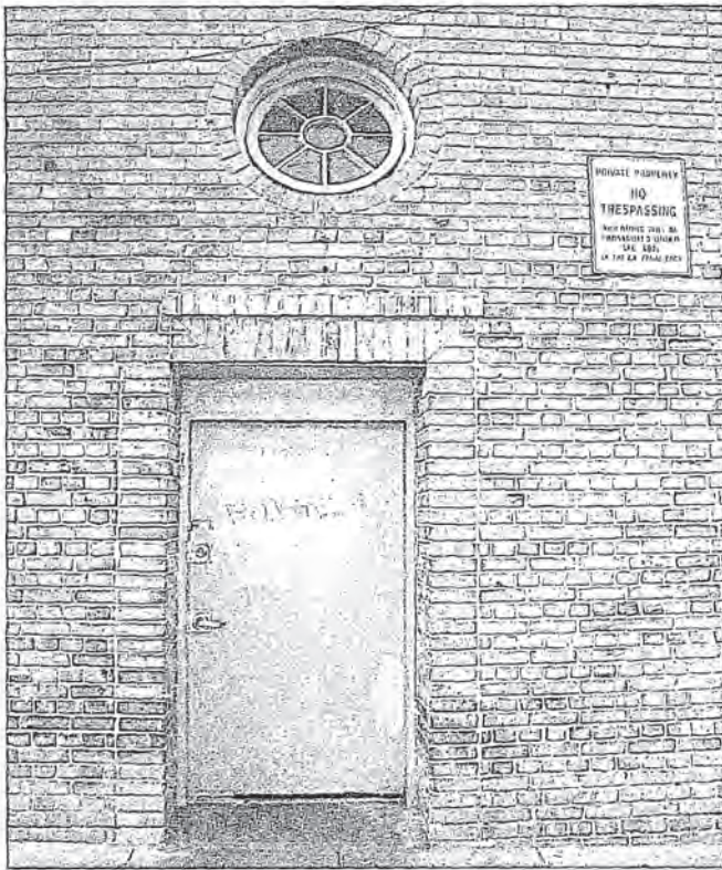
Photo 6. August 2007. Cambridge Apartments, Commercial Entry, North Façade.
