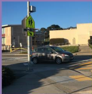
RECTANGULAR RAPID FLASHING BEACON
