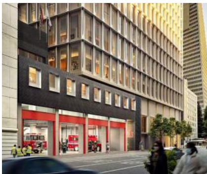
Fire Station 13, San Francisco, CA
