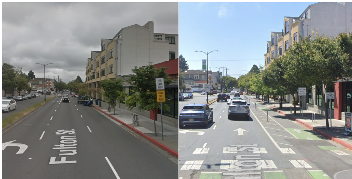
Before-and-after comparison showing the quick-build bicycle facility constructed on Fulton St. in 2016 (Google Street View).
