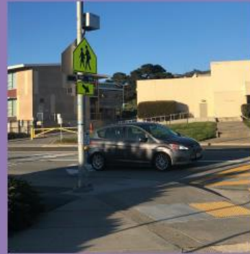
RECTANGULAR RAPID FLASHING BEACON
