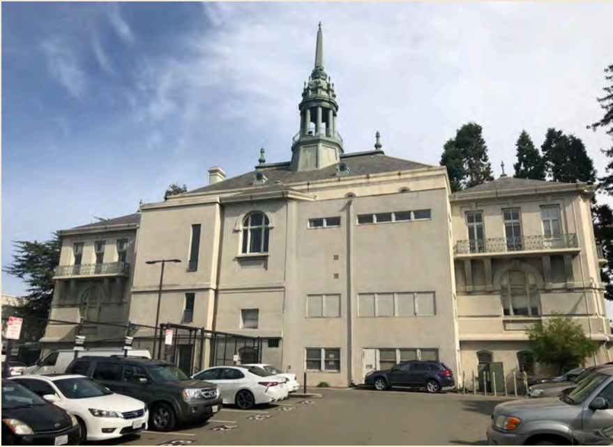
Figure 6.13 West (rear) façade.
