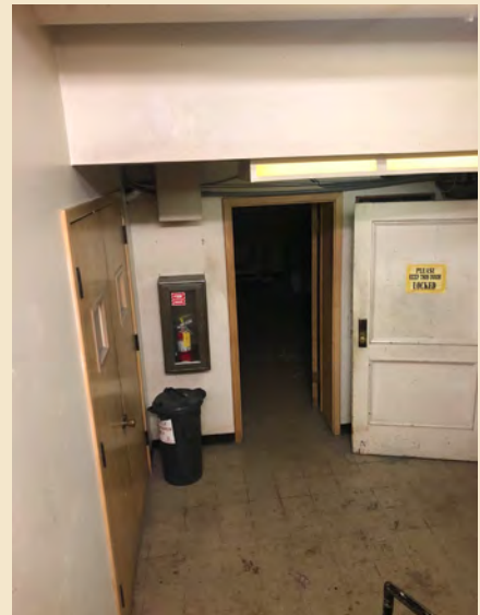
Figure 6.30 Remnant paneled wood door in basement.
