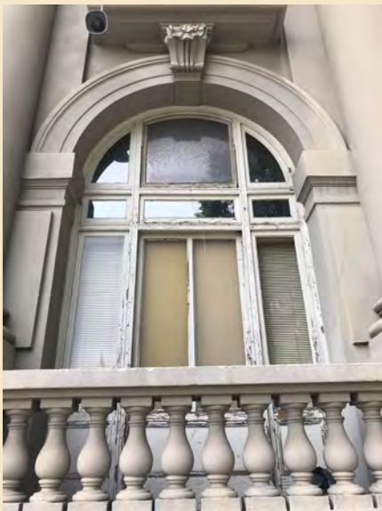
Figure 6.15 Semicircular-arched window with pronounced springers and ancon and swag keystones are found throughout the building.
