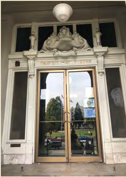
Figure 6.8 Original main entrance surround with modern replacement doors.
