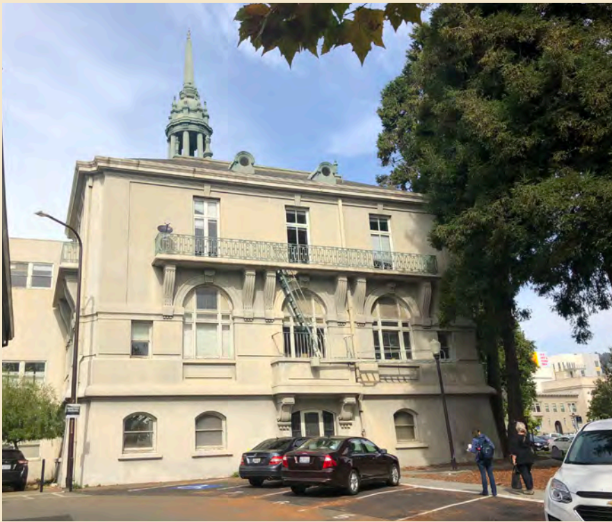
Figure 6.10 South (side) façade.
