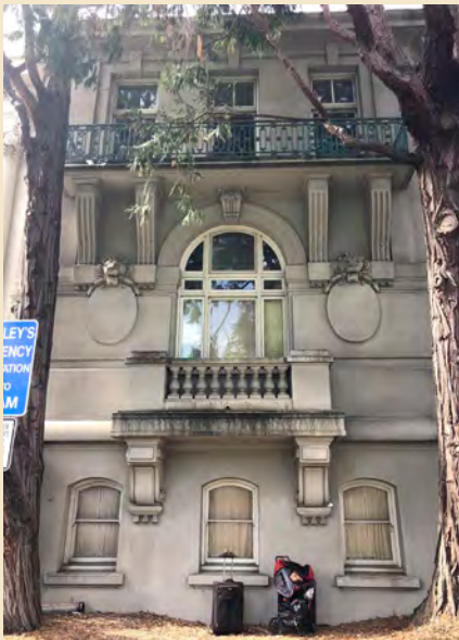
Figure 6.9 East (front) façade of the south wing.
