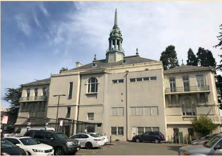
Figure 7.4 The original stair tower of the rear (west) façade has been engulfed by two additions, rendering the historic façade unreadable.
