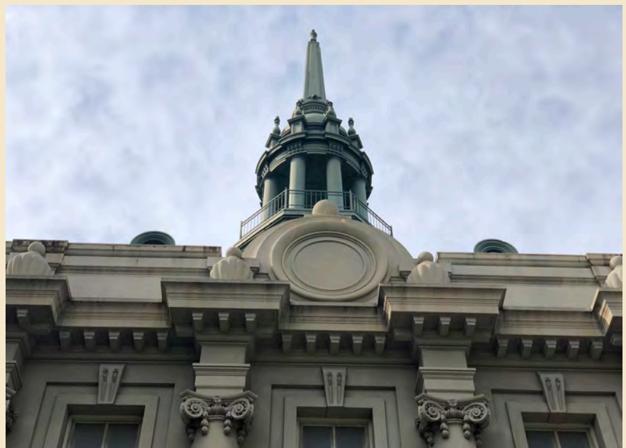
Figure 6.6 The octagonal cupola and spire are made of sheet metal on a wood frame.
