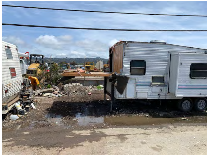
2 nd and Jones (Unsafe Structure)- After
