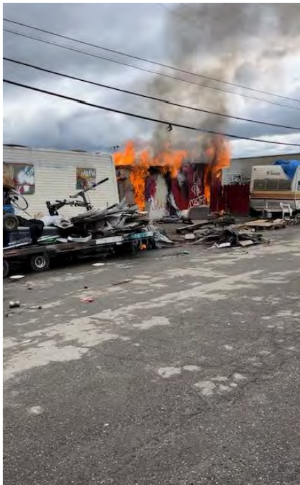
2 nd Street – Structural Fire
