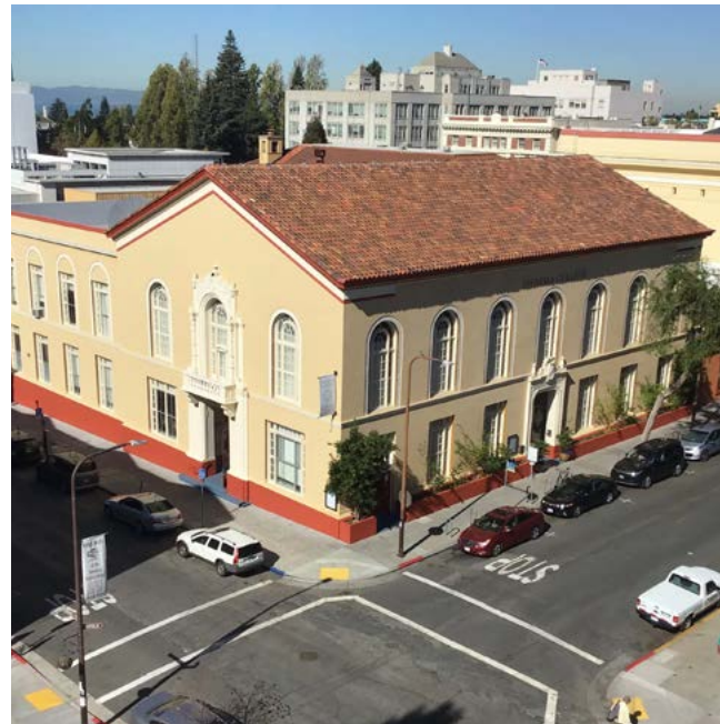
Dharma College is now located in the former Armstrong Business School Building
