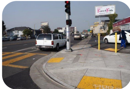
ADA ramp and signal upgrades
