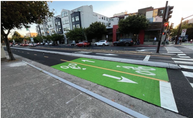
Figure 6 Two-way protected cycletrack on Fulton St in Downtown Berkeley. Cycletracks (class IV bike facilities), like those recently constructed in Downtown Berkeley, would be key for the Waterfront’s long-range reduction in single occupancy vehicle trips. (Source: Jonathan Zisk)
