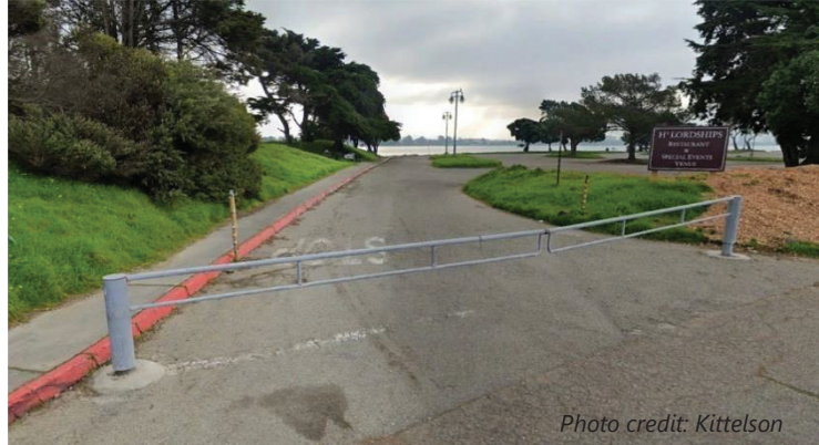
Figure 11: Gates at Seawall Drive Lot
