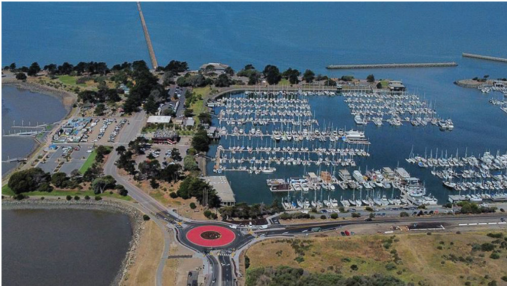
Figure 3 Parking facilities currently occupy 20% of the Waterfront’s in-demand space for natural recreation. Right-sizing and regulating parking facilities is a critical step in preserving both natural resources and visitors’ access to them. (Source: City of Berkeley, Waterfront Specific Plan (Draft) , 2023.)
