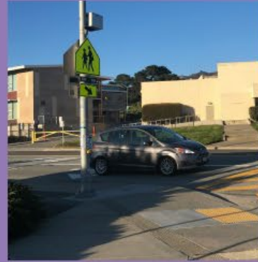
RECTANGULAR RAPID FLASHING BEACON
