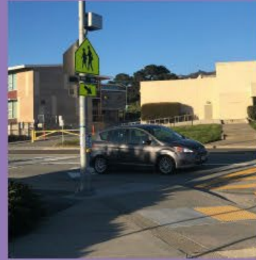
RECTANGULAR RAPID FLASHING BEACON
